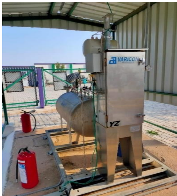
(Figure: 5 Odorization Unit)
