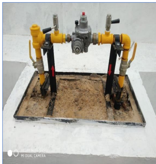
(Figure:7 Service Regulator)
